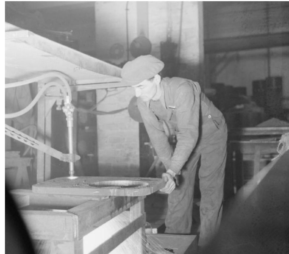
← Tyneside Ship-yards, 1943 A man cutting circular steel plates at a machine.
