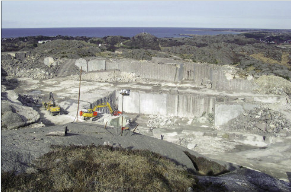
Anorthosite quarry at Sirevåg, Rogaland (Photo: T. Heldal)
