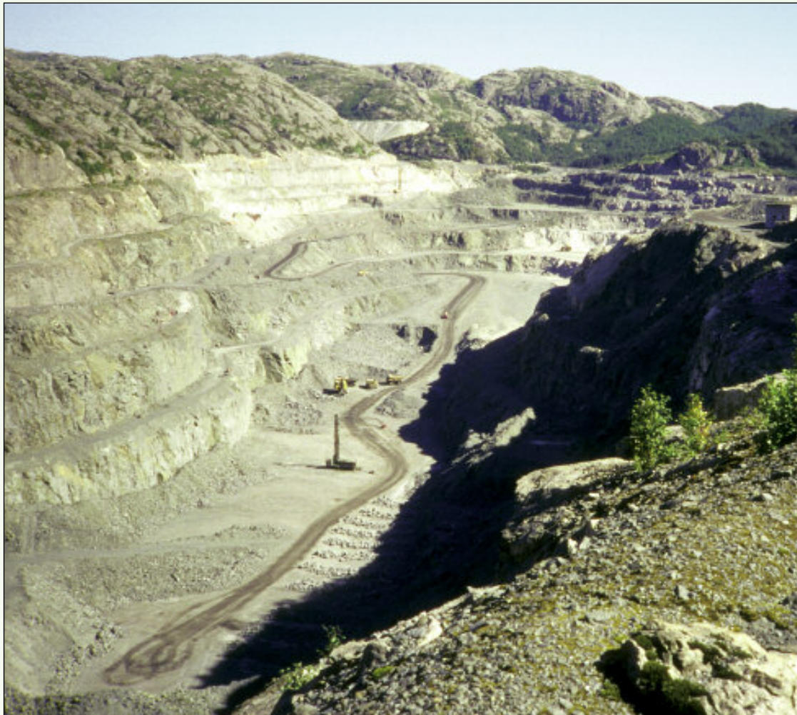
Opencast mine at Tellnes, Sokndal, Rogaland, where Titania AS works ilmenite ore. (Photo: L.-P. Nilsson)
